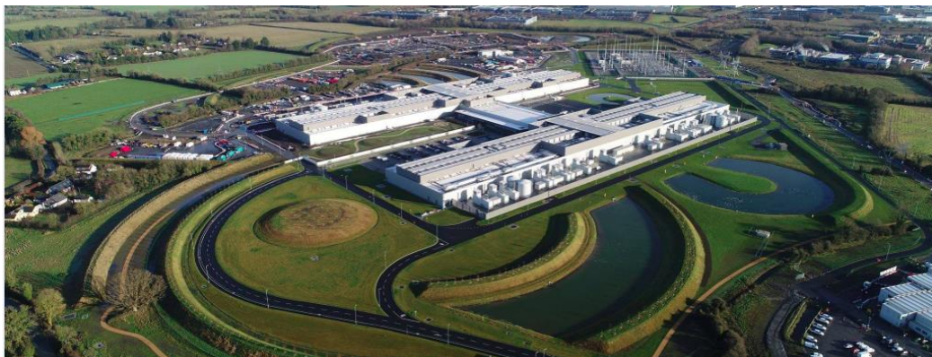
Facebook Data Centre at Clonee, Co. Meath with associated electrical transformer infrastructure top RHS
